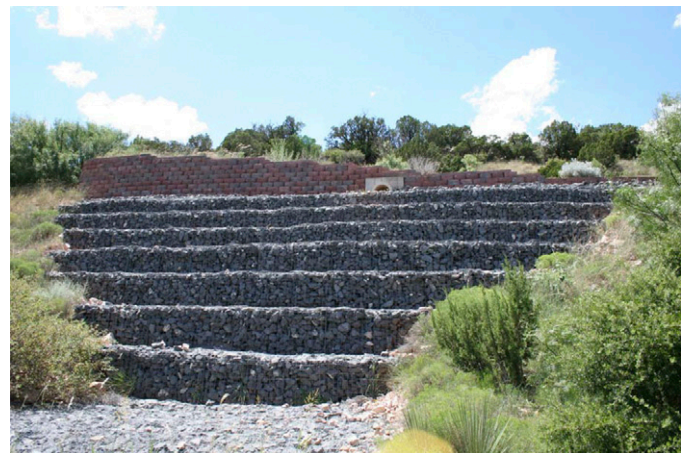
Fig. 4. Gabion and outfall
