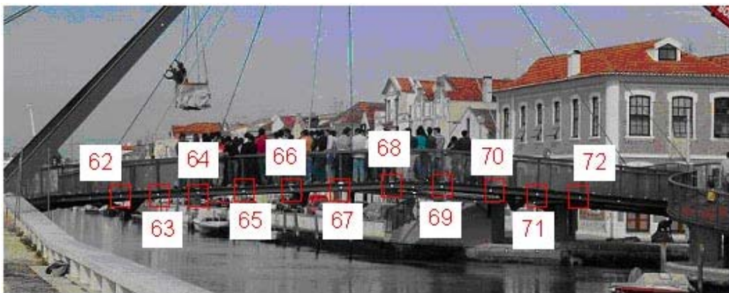
Fig. 8 Vertical displacements for SE loading situation.
